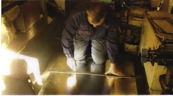
Marking the sheet for the height of the cylinder
