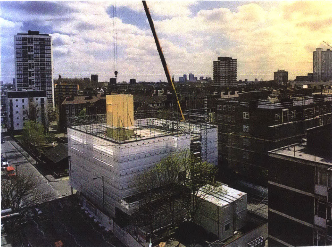
Note CLT elevator shaft. Source: (Ibid, pp. 41)
