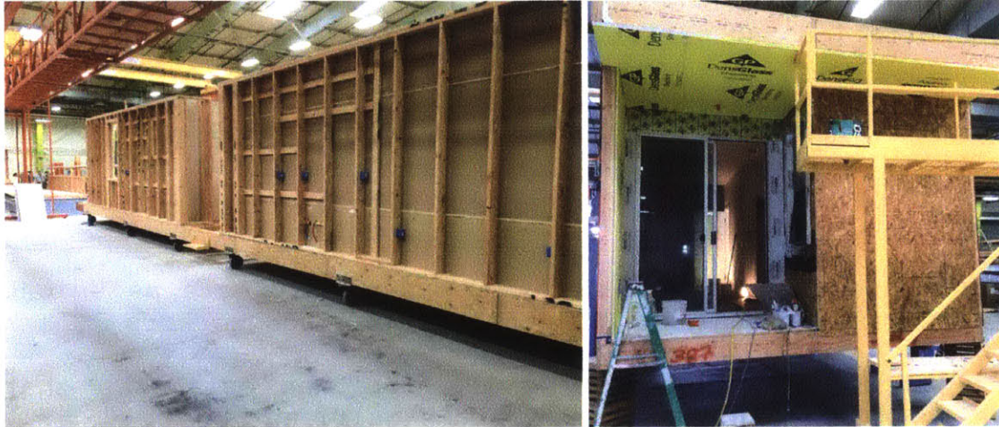
Figure 9 - FBH Modules Under Construction
