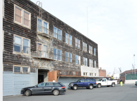
Building 11: The Noonan Building “Context Resource” to be demolished. 33,000 sf; wood frame; built 1941
