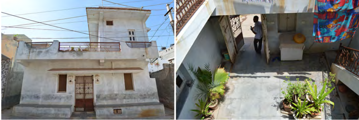
Figure 3.6 – Exterior images of Building 3. Left: View of the north facade. Right: View into courtyard during mid-day.
