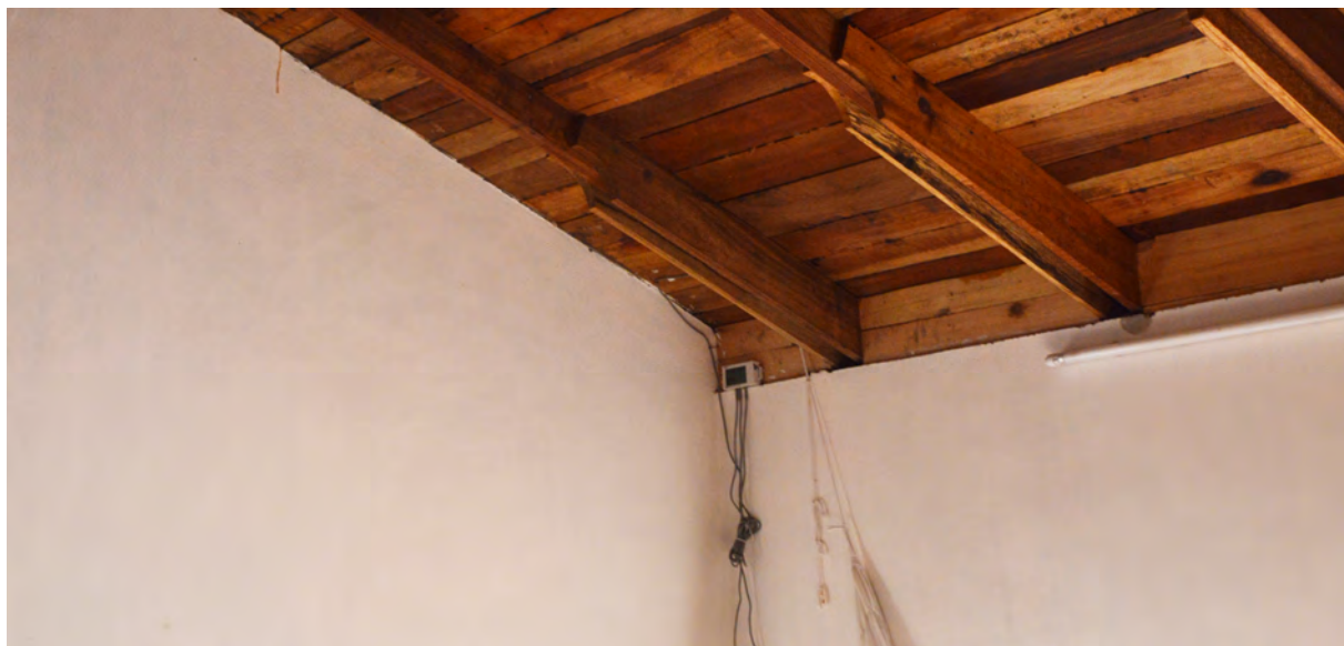
(b) Interior of Building 2 Showing Ceiling and Wall Materials.
