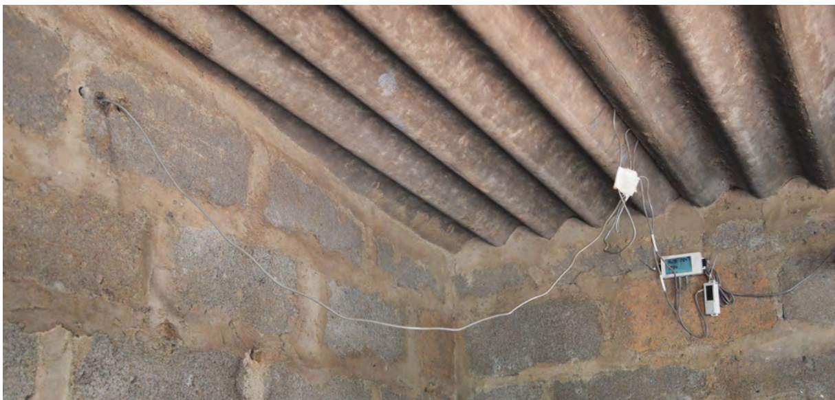
(b) Interior of Building 1 Showing Ceiling and Wall Materials.
