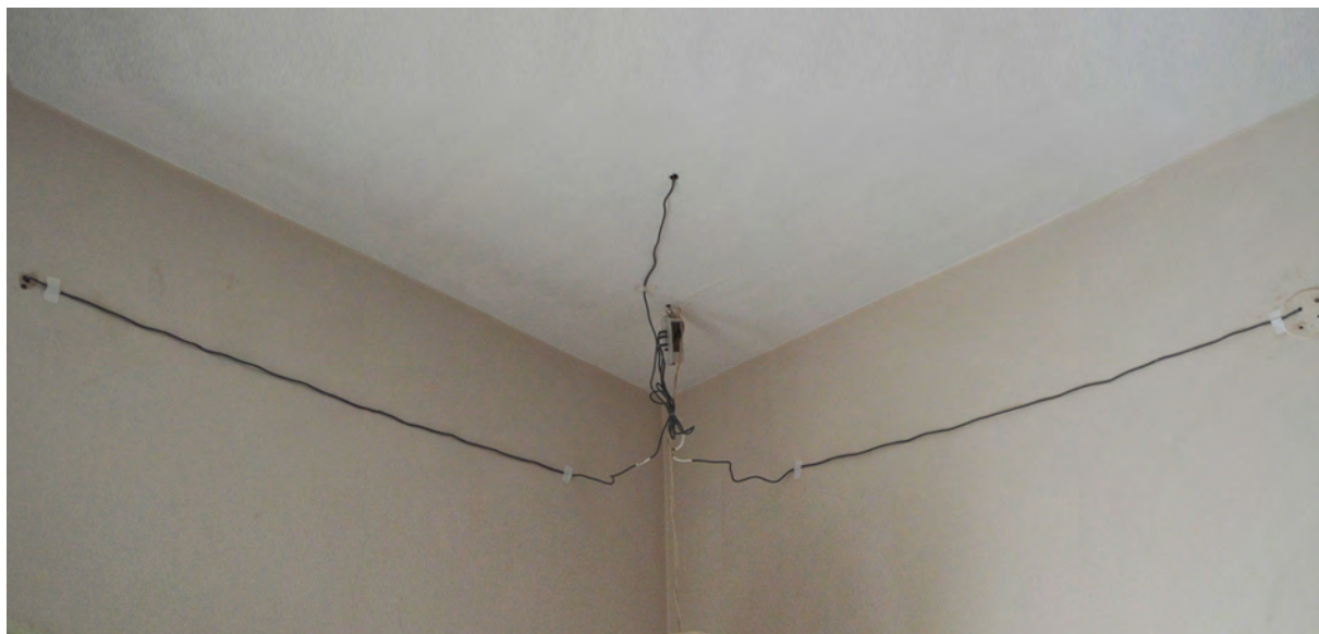
(b) Interior of Building 4 Showing Ceiling and Wall Materials.
