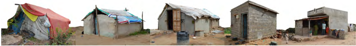
Figure 2.7 – Common Bhuj Informal Housing Construction Types. Examples of temporary to more permanent construction types are pictured from left to right.
