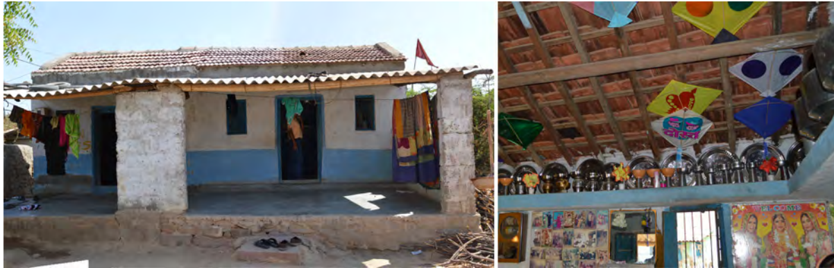
Figure 3.21 – Images of Building 6. Left: View of the south facade. Right: Interior view of uninsulated Mangalore Tile roof.
