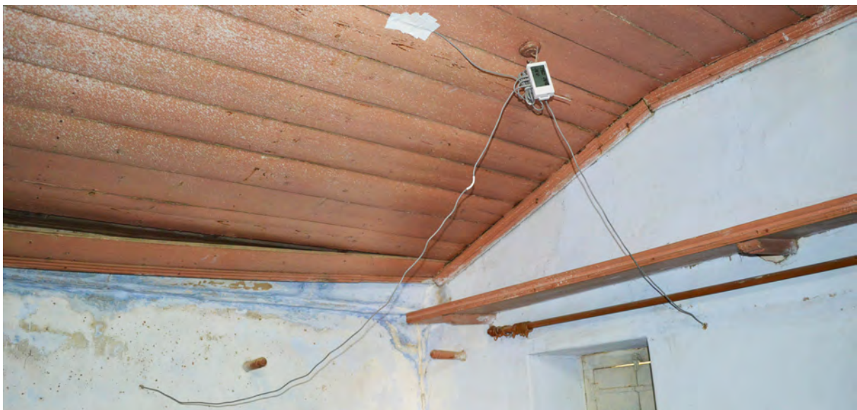
(b) Interior of Building 3 Showing Ceiling and Wall Materials.
