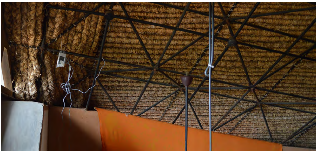
(b) Interior of Building 5 Showing Ceiling and Wall Materials.
