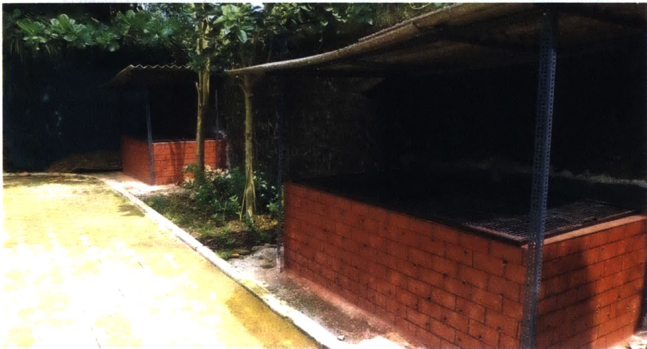
Figure 12: Onsite Composting Pits at Institution (Banerjee 2015)
