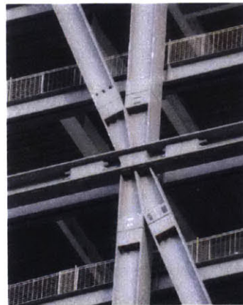
(b) Steel Customized Plate Node
