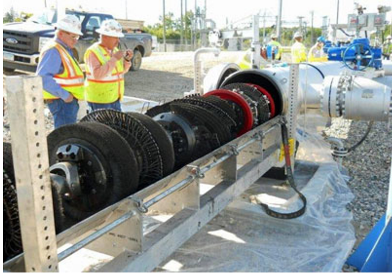
Figure 1-1: ILI Tool being loaded into a pipeline [Offshore Mag., 2012]
