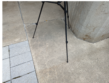
(g) O3 measuring concrete surface material
