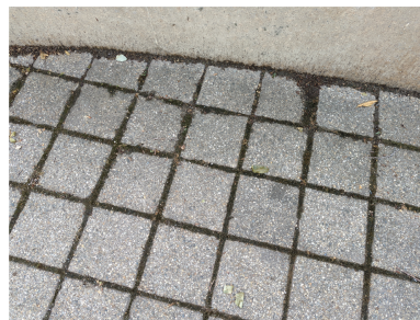
(g) MM3 measuring paver surface material
