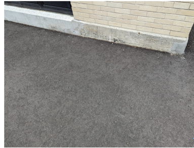
(c) O1 measuring asphalt surface material
