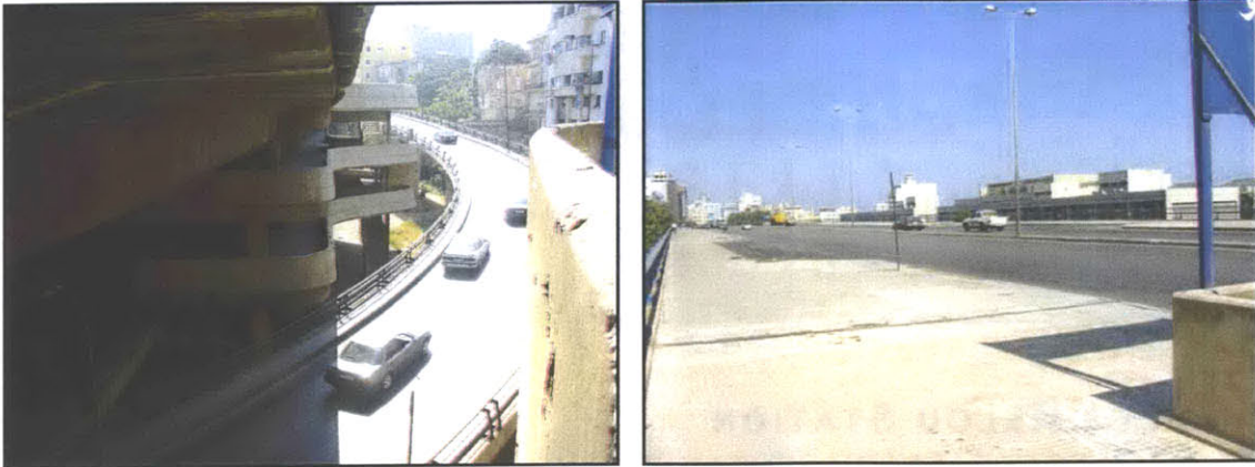
Figure 4-6. Charles Helou Avenue viaduct
