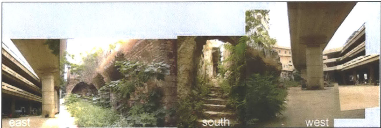
Figure 4-8. The south side of Charles Helou Station
