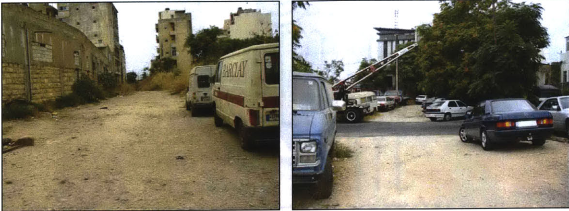
Figure 4-14 (A and B). The ramp into the tunnel is overgrown and has been used for dumping; a single narrow/wide gauge track remains inside the tunnel
