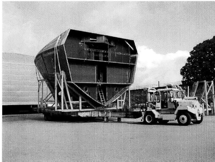
Figure 14: Bow section of the Visby-class corvette under transportation to the outfitting workshop. [Ref 103]
