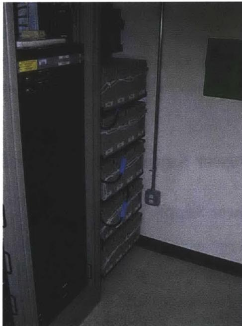
**Figure 1.3 VRLA Battery bank in NEXTEL base station, Green St., Cambridge, MA**
