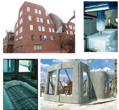
Figure 1.1 Fabrication of Styrofoam molds PROJECT: Case Western Reserve University LOCATION: Cleveland, Ohio ARCHITECT: Gehry Partners
