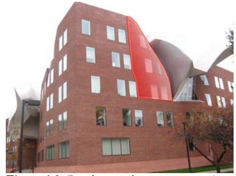
Figure 1.0 Complex-curved masonry construction PROJECT: Case Western Reserve University LOCATION: Cleveland, Ohio ARCHITECT: Gehry Partners
