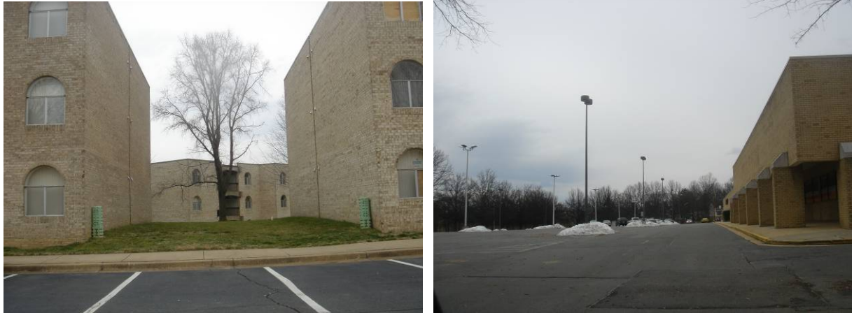
Proposed suburban retrofit in Tysons Corner, VA. Includes a declining apartment complex and failed retail mall. Source: Amy Merritt
