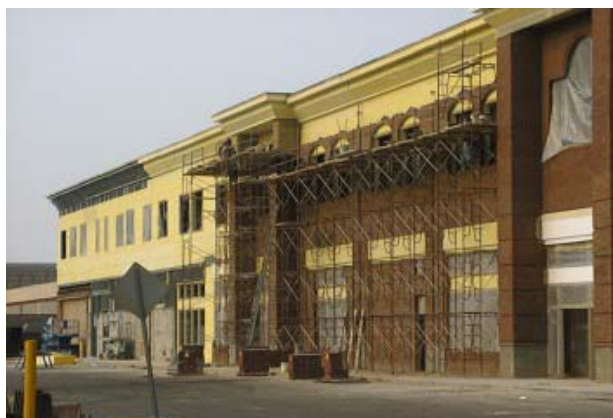
Eastgate Mall under construction, 1998
