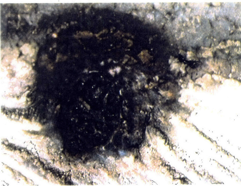
Figure 7.2.2. Surface discontinuity (inclusion) at weld edge of MT-3
