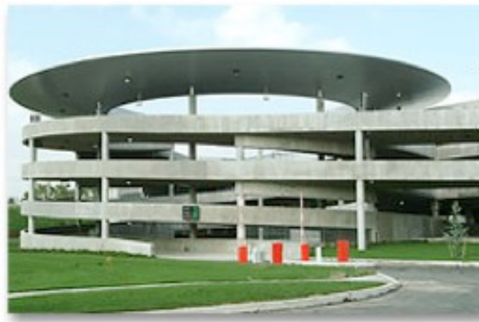
Figure 4.1: Example of parking garage. (Source: SARAA, 2007).
