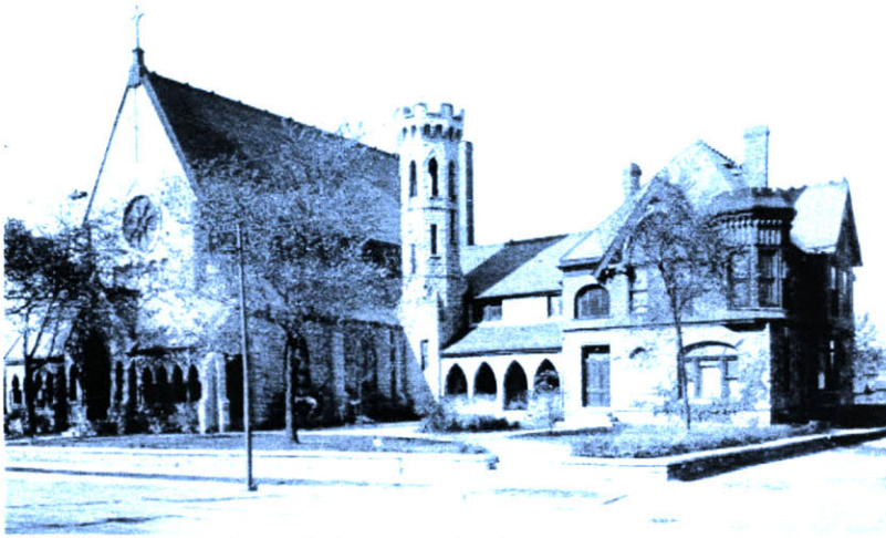
4.6 1917 view of the historic Christ Episcopal Church.
