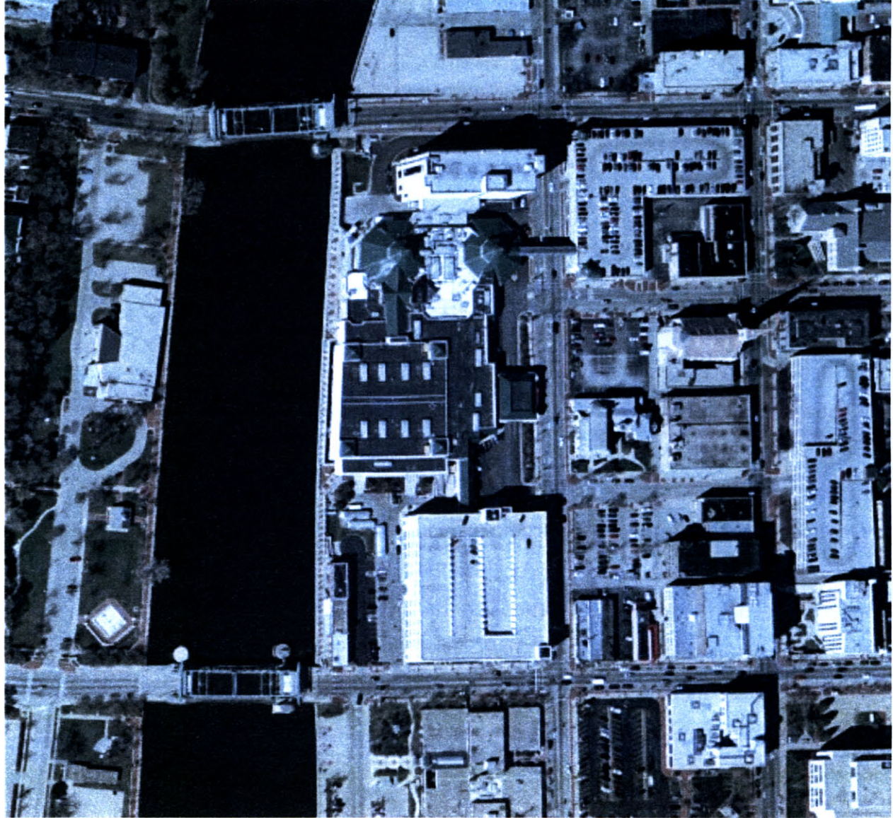
4.2 Aerial view of Harrah's Joliet Casino.
