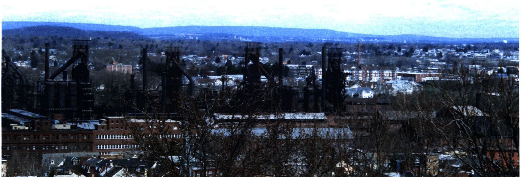
1.2 South Bethlehem Blast Furnaces
