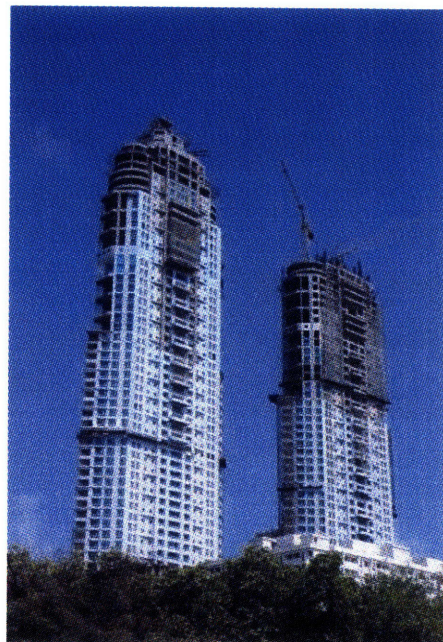
HIGH RISE CONCRETE FRAMES ON THE MILL LANDS - ADVENT OF A NEW RESIDENTIAL FACADE IN THE FORM OF GLAZING
