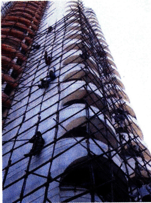
EXTERNAL PLASTER MASONS
