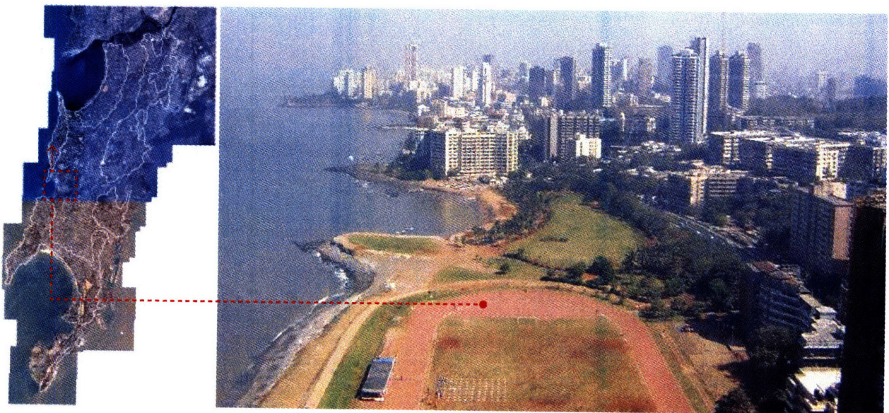
LOOKING NORTHWEST FROM MAHALAXMI RACE COURSE [ON RECLAIMED GROUND] TOWARDS THE ISLAND OF WORLI
