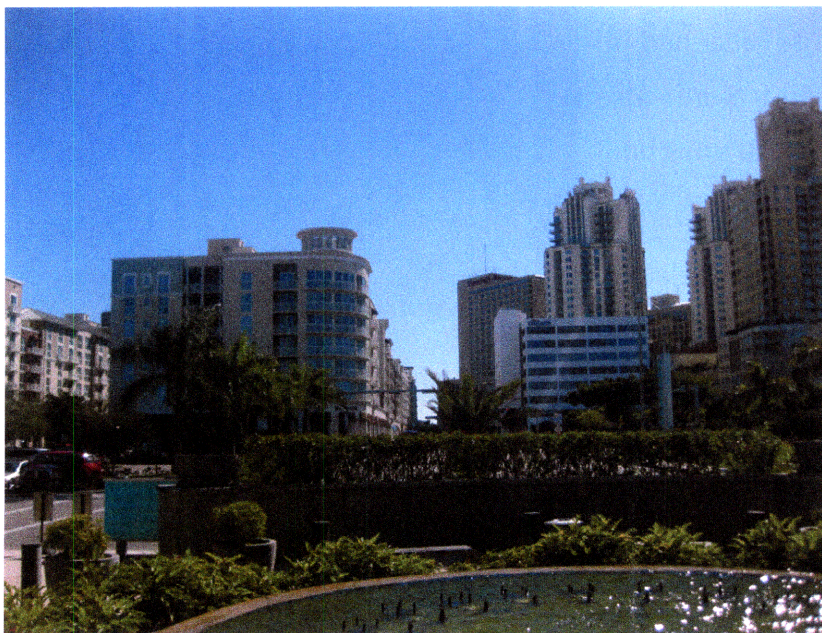
High-density buildings in the Downtown Kendall TODs as viewed from Dadeland Mall.
