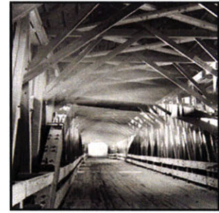
Fig. 163 Covered bridge in Vermont, from [125]
