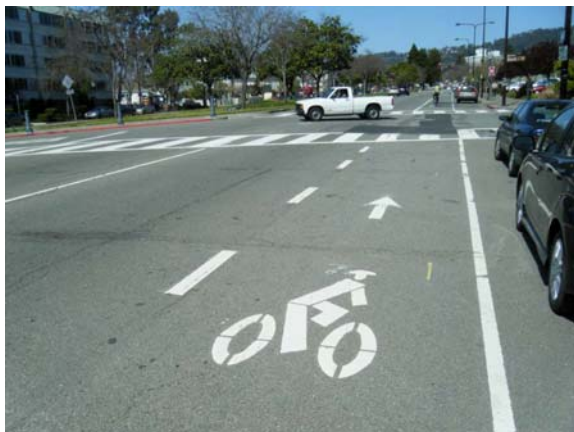
Figure 24. Bike lane on Adeline St.
