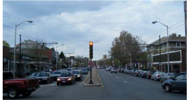
Figure 43. Mass Ave. parallel to Oxford St.
