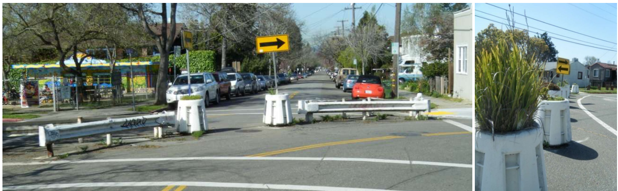
Figure 16. Guard rail diverters on Virginia St. (left) and flowerpot diverters on Ninth St. (right)
