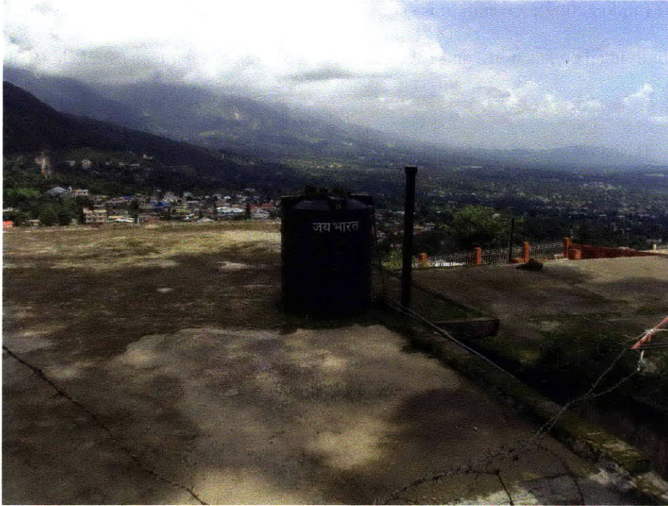
Figure 6: A Roof-top Storage Tank in a Household with a Private Water Connection
