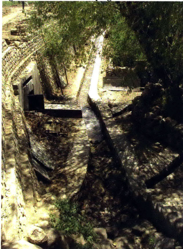
Figure 18: Channel conveying Water from Pond to Farmlands
