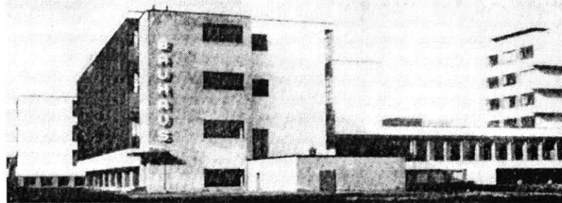
Figure 2.11: The Bauhaus at Dessau, designed by Walter Gropius, 1926
