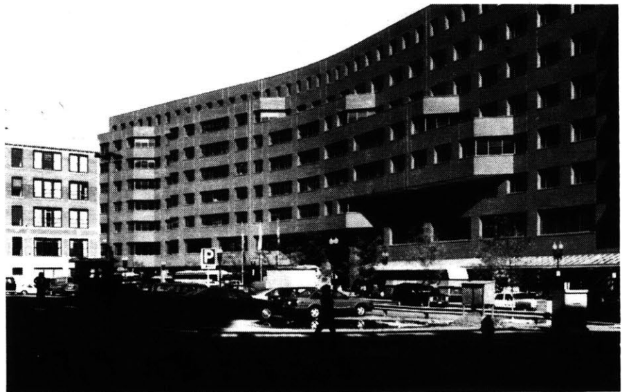
Figure 4.11 The site (at left foreground), and the State Transportation Building, viewed from across Tremont Street looking northwest.
