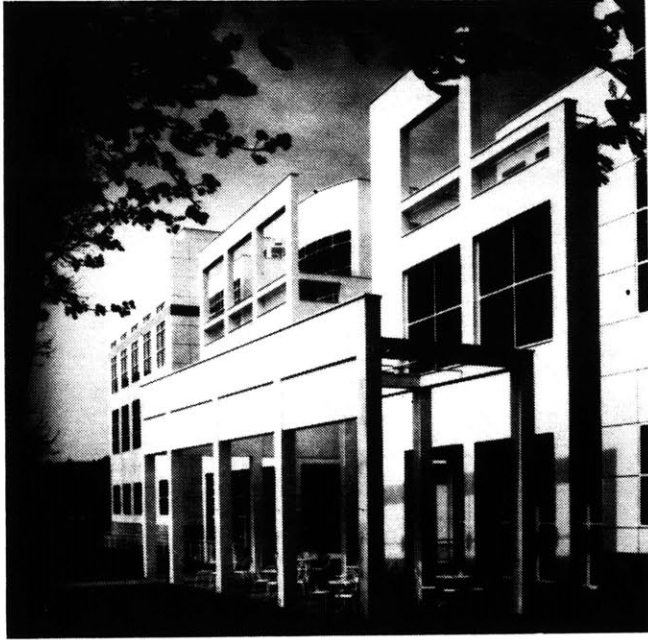
Figure 6.18 Meier's Frankfurt Museum employs screen walls to break down the mass of the building and to create a layering of spaces around it.
