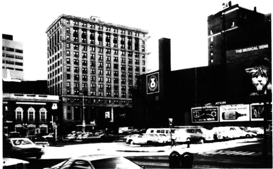
Figure 4.9 The site, viewed from across Stuart Street, looking southeast.
