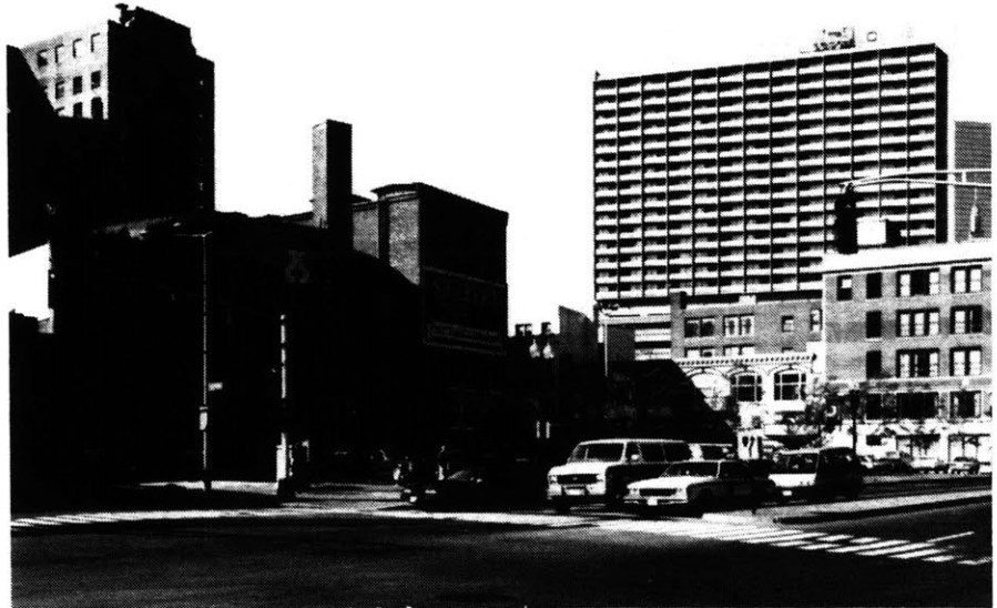
Figure 4.10 The site, viewed from the corner, looking southwest.
