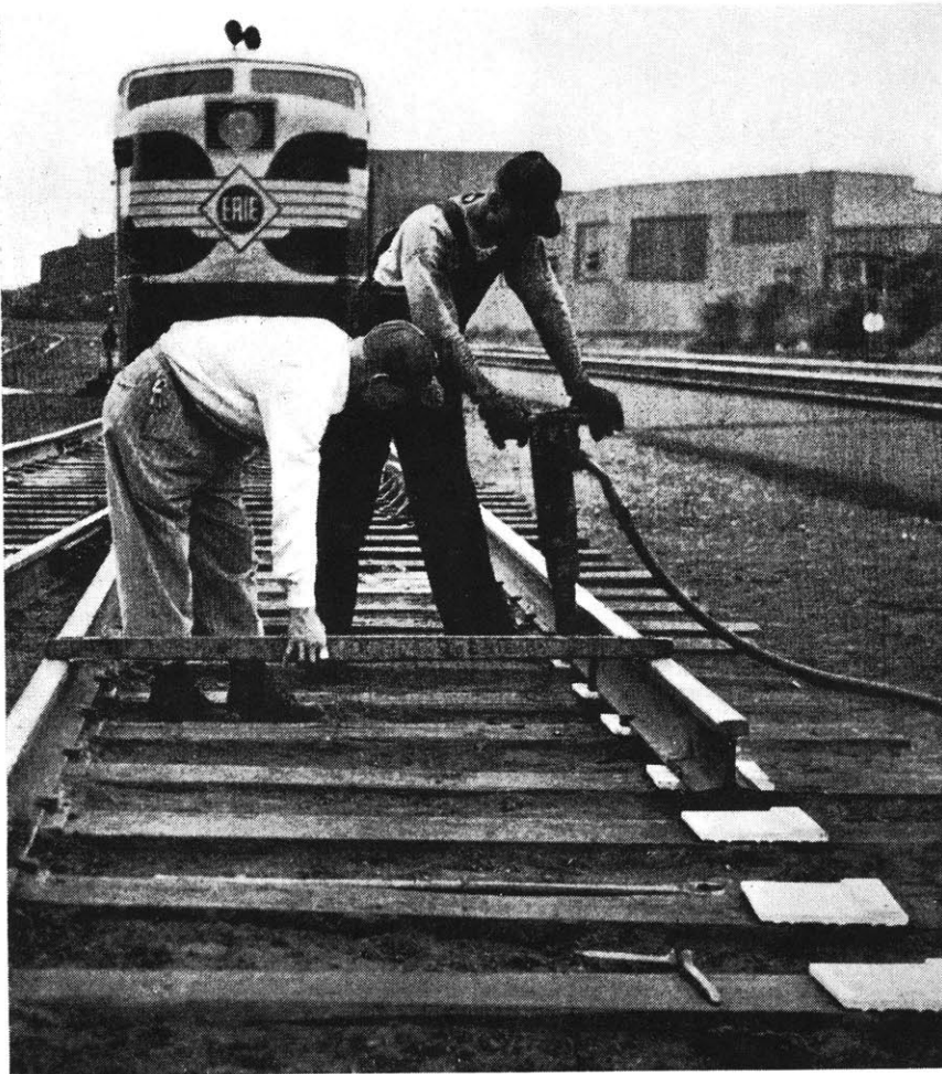
Glass-reinforced polyester track rail support plates have the required strength, corrosion resistance and resiliency. (Dynakon Corp.)
