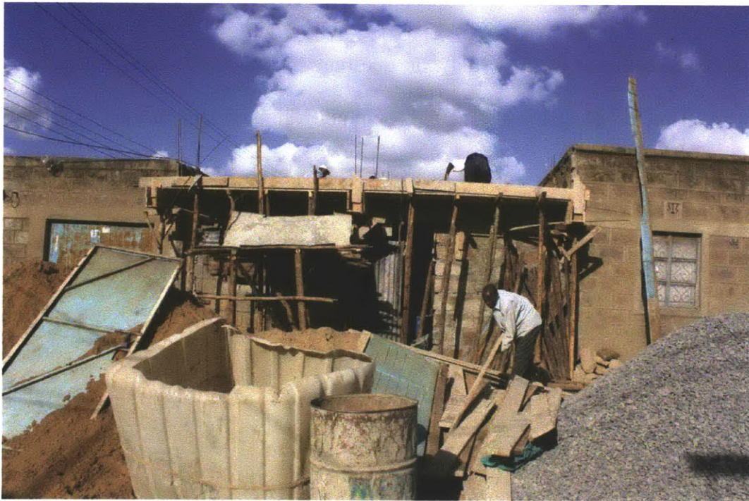
FIGURE 4.4: Do It Yourself (DIY) construction in Dandora, Kenya (2010)
