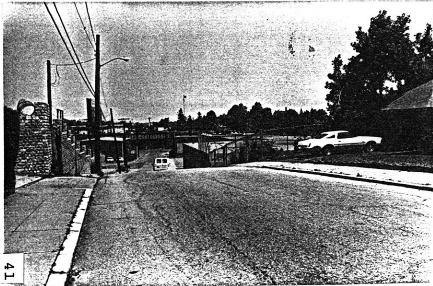
41 Good Enough Street, looking north to Mass Pike.
