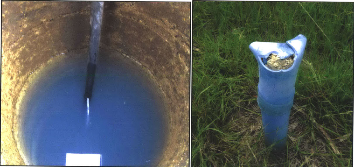
Figure G-1: Left, turbid but better tasting borehole in Duuyin; Right, Tugu borehole was sealed because it produced salty water that was considered unfit for human consumption.
