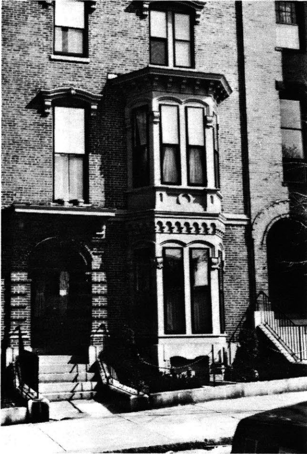
Figure 7-7. 12 Monument Square, facade detail.
