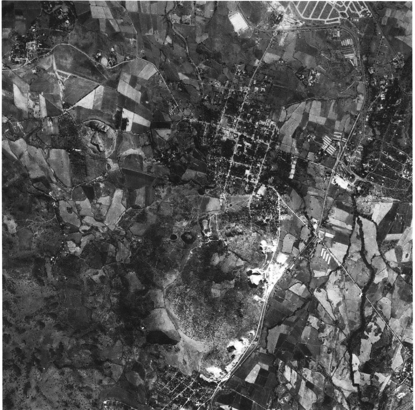
The aerial photograph shows the layout of the town of Jiutepec and the surroundings. Its limits to the north is a textile factory and a cement factory; to the south: idle lands, the site that is proposed, and lime stone quarries; to the east high income developments for weekend houses. To the northwest and southeast are irrigated agricultural lands. The scale is 1: 20000, the same as the plan in the opposite page.
