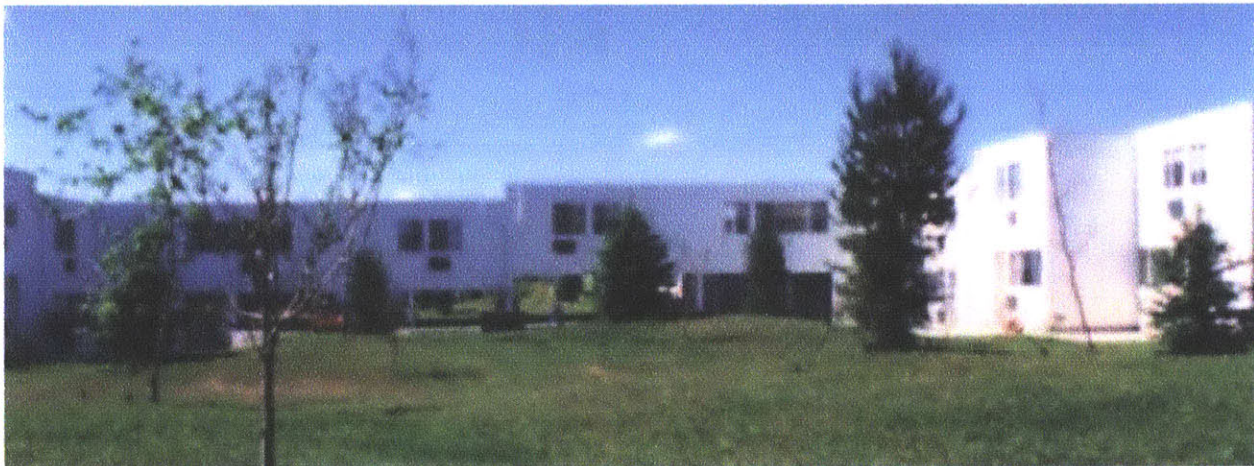
Figure 5.2 : Two views of Pines of Perinton development, designed by Gwathmey Siegel. 2004 | Source: Policy and Design for Housing: Lessons of the Urban Development Corporation 1968-1975. Part 1.
