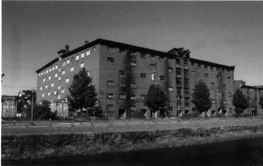
Existing Mill Building Exterior.
