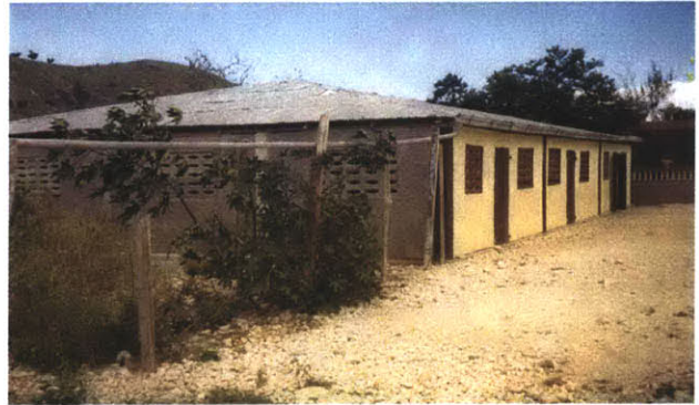
Figure 6.9: Roof Draining to Cistern
