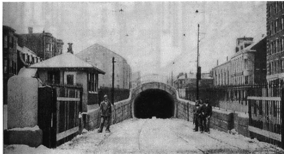
image 12. The East Boston Tunnel entrance from Maverick Square, 1905
