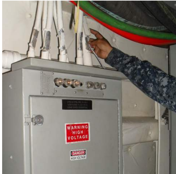
Figure 5-3: Sailor Holding Non-Contact Sensor to Power Cable on NEW ORLEANS
