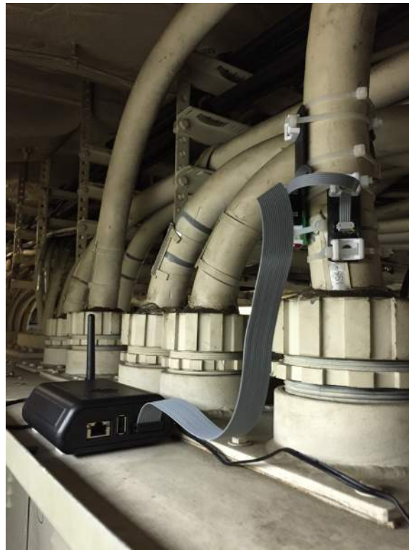
Figure 5-4: Non-Contact NILM Installation on USS CHAMPION (MCM 4)
