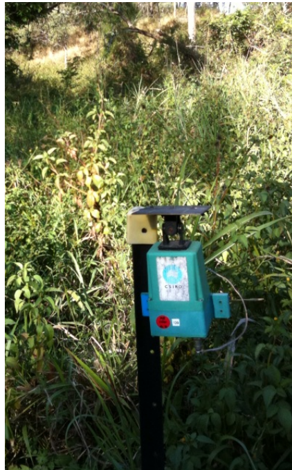
Fig. 1. Fleck Node Installed on Campus
