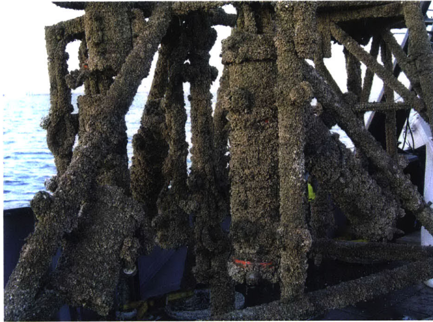
Figure 4-1: After several months of exposure to marine life, heavy biofouling develops on offshore structures. Such biofouling is an obstacle to thorough inspections and non-destructive testing [54].
