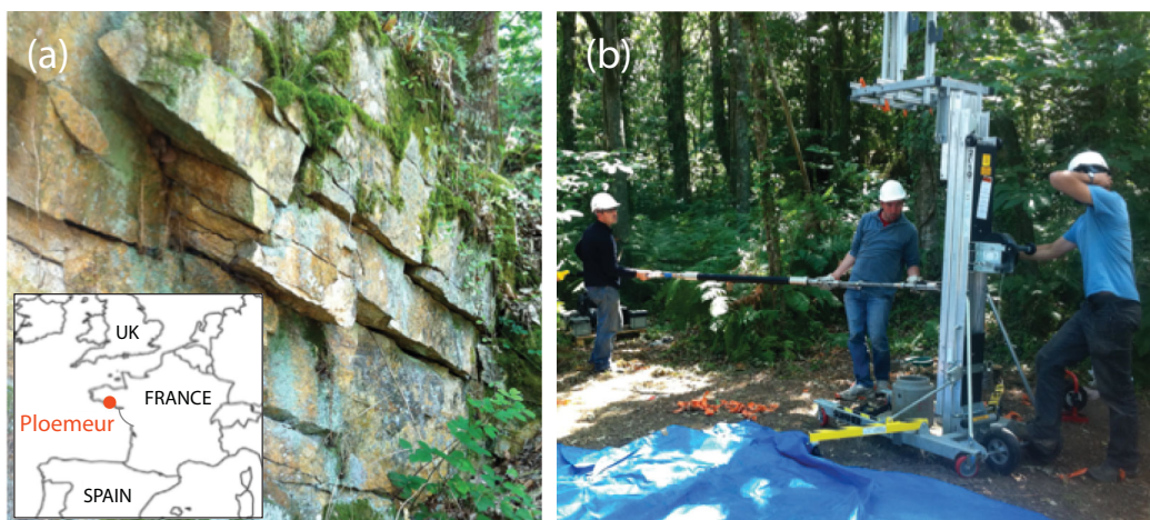
Figure 1. (a) Outcrop of fractured granite at the Ploemeur field site. Inset: map showing the location of Ploemeur, France. (b) Photo from the installation of double packer system in B1 borehole.
