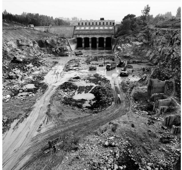
Reservoir for South to North Water Transfer Project under construction
