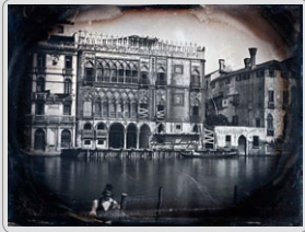
Daguerreotypes of The Grand Canal. The Casa d'Oro Under Restoration, John Ruskin
