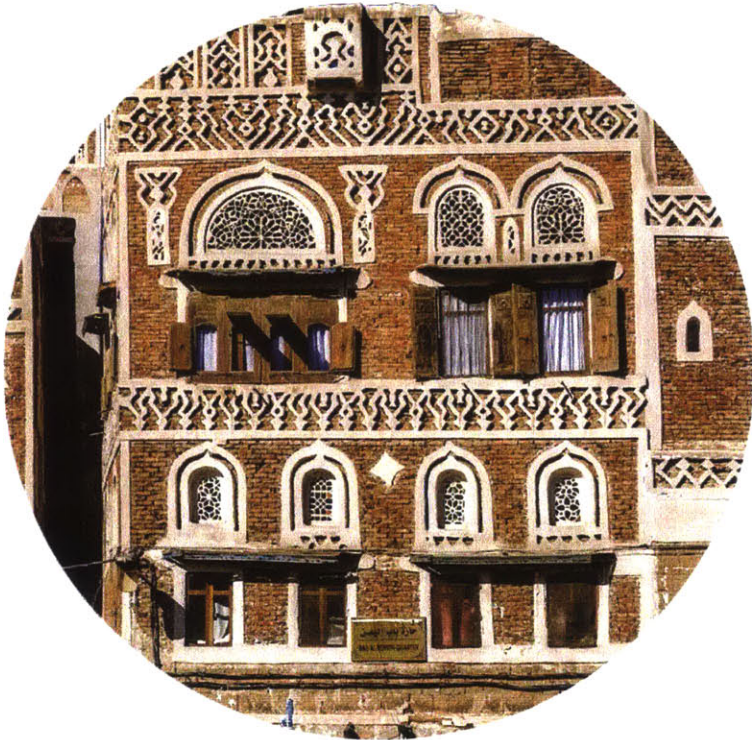
Plaster Window Ornamentation
