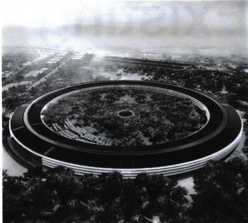
Apple Headquarters - Mountain View, CA - Under Construction
