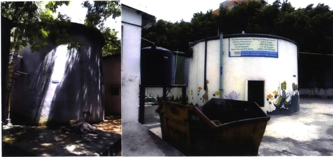
Figure 54: Five-ton per day anaerobic digesters in Pune.
