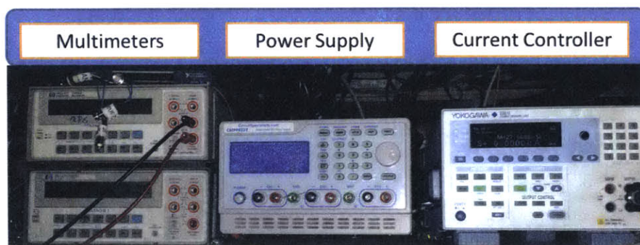
Figure 5-10: Image showing the control devices used to perform the measurement.
