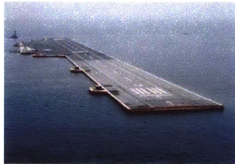
(b) 1000m long Mega-Float in Tokyo Bay (a test for a floating airport) (Wang and Tay, 2011)
