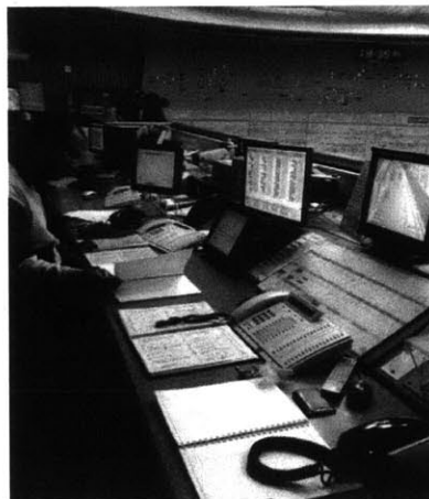
Figure 2-10: Earl's Court's controllers desk
