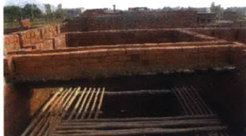
3 BRICK MASONRY IS DONE AS FORMWORK. CLAY IS USED AS MORTAR.
