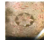
DOME WHEN THE SHUTTERING IS REMOVED IN 19 DAYS AFTER CASTING.
