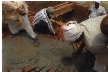
CONCRETE IS MANUALLY PUT BETWEEN THE BRICKS AND SMALL GAPS
