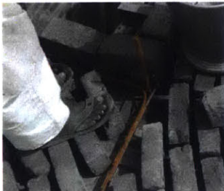
AT T JUNCTION WITH OVERLAPPING BAR
