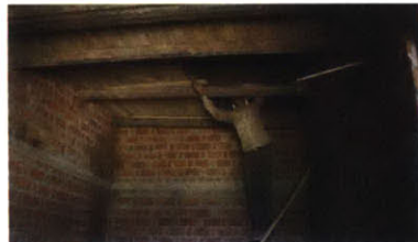
THE PLANKS ARE REMOVED FIRST.
