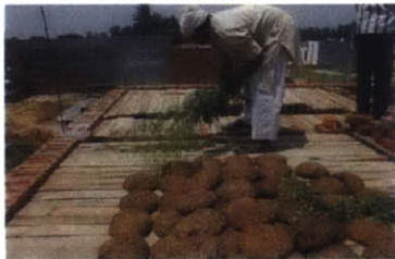
THE GAPS IN THE PLANKS ARE FILLED BY BUSHES.
