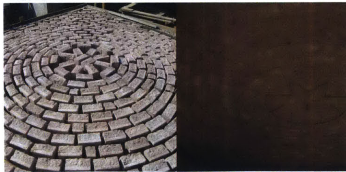
Shallow Dome Built At Hunnarshala
