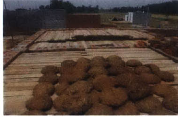
DUNG CAKES ARE USED TO GIVE THE BASIC DOME SHAPE. THE MAIN ADVANTAGES OF USING THEM ARE THEIR LIGHT WEIGHT AND RE-USIBILITY.
