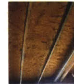
DOME WHEN THE SHUTTERING IS REMOVED IN 10 DAYS AFTER CASTING.
