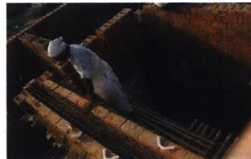
4 REINFORCEMENT IS PLACED AND CONCRETE IS POURED
