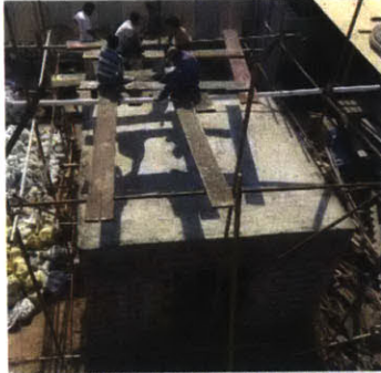
Scaffolding is Prepared For Loading
