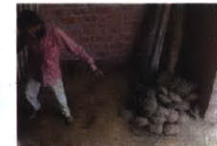
DUNG CAKES USED IN FORMWORK ARE REUSABLE.
