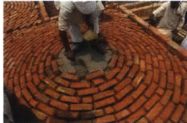
CONCRETE IS MANUALLY PUT BETWEEN THE BRICKS AND SMALL GAPS
