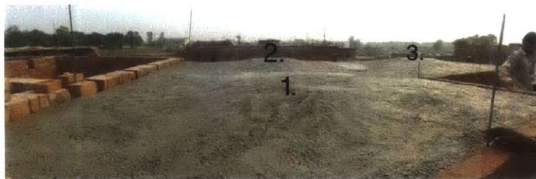
DOMES 1, 2 AND 3 AFTER THE CONCRETE IS POURED.
