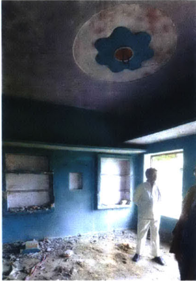
AFTER THE CEILING IS PLASTERED AND PAINTED, AT KUTBA VILLAGE, MUZAFFARNAGAR
