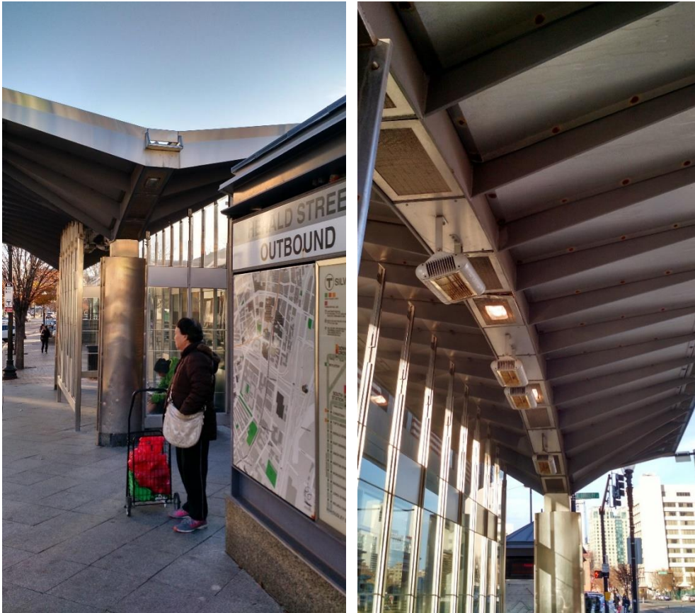
Figure 5.8 - Silver Line stop infrastructure on Washington Street
