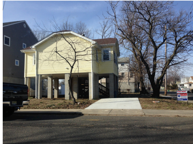
Fig. 4-18: One of many homes raised above flood levels in Keansburg's coastal neighborhoods.
