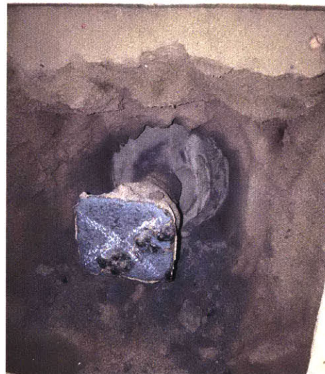
Figure 33: Excavating the piston.
