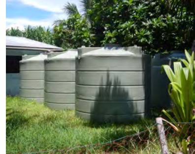
Water tanks outside a home on Funafuti. Rainwater is the primary source of water for drinking, washing, and bathing in Funafuti as well as some outer atolls which have damaged freshwater lenses. In Funafuti, these tanks encroach on valuable real estate, and homes increasingly utilize 2 or more tanks.
