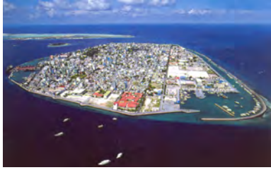
Male, Capital of the atoll nation of the Maldives. Fortification and land-building processes have eliminated this atoll's ability to respond to sea level rise through coral/atoll processes. Source: Wikimedia Commons
