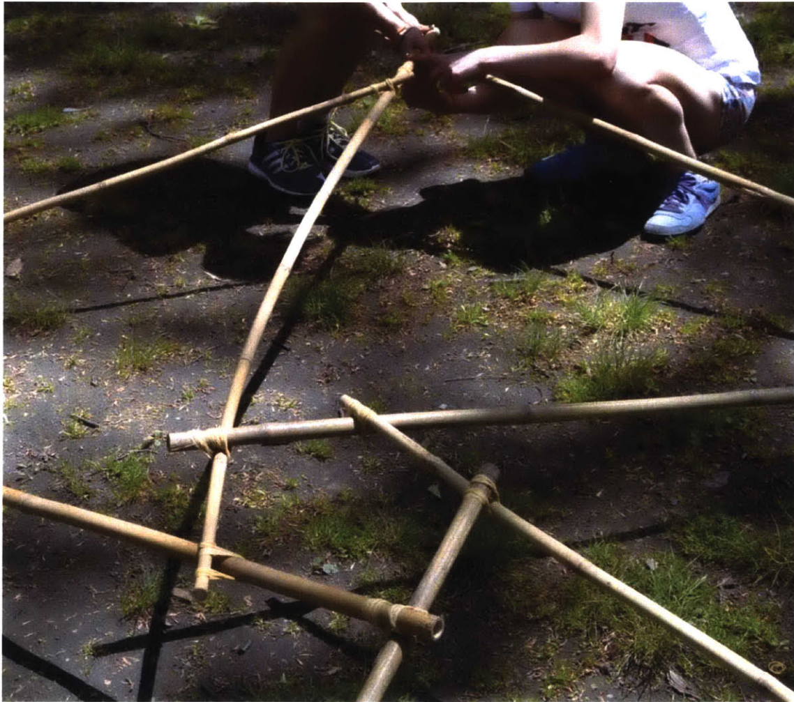
Figure 4-18: Photograph to show bamboo bowing.
