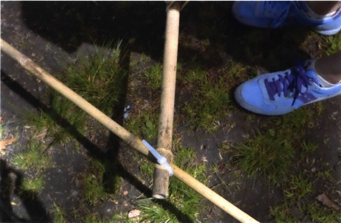
Figure 4-20: Zip tie preventing joint movement.
