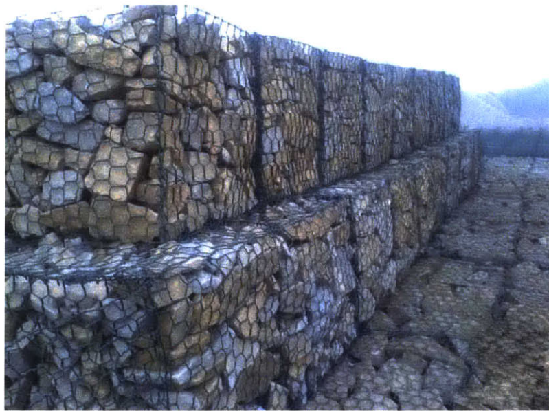
Figure 4-5: Photo to show gabions [7, Nitin Wirenetting, 2015].
