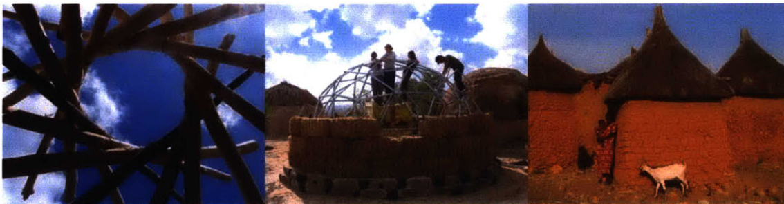
Figure 4-2: Left: Example of a reciprocal joint [18, Lewandowski, 2015]. Center: Geodesic dome home construction in Israel [15, Dodinval, 2015]. Right: Mud and straw houses in Sudan [20, Mysliborski, 2006].
